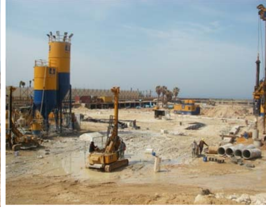
Figure 8: Equipment at working platform Figure 9: Drilling of grouting holes
